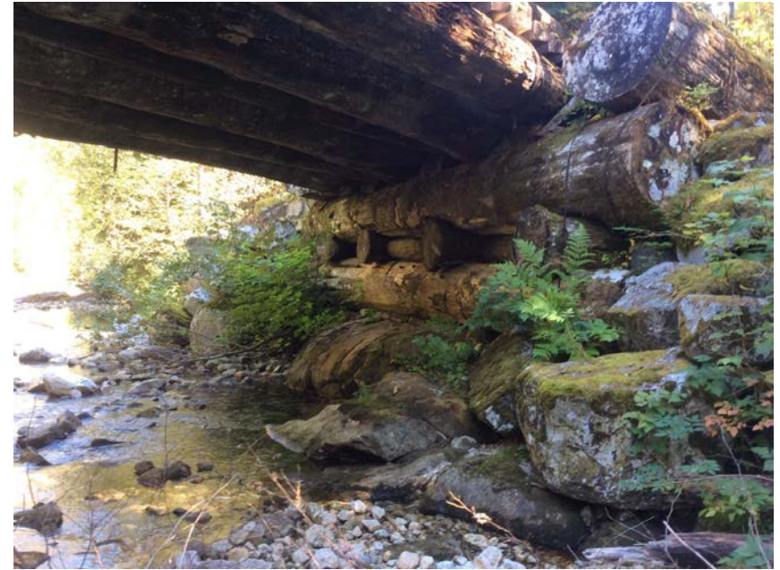
Right Bank Abutment when facing downstream
