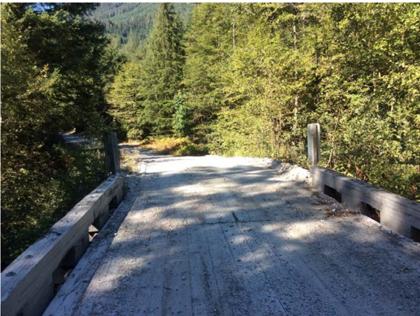
Left approach viewed from bridge
