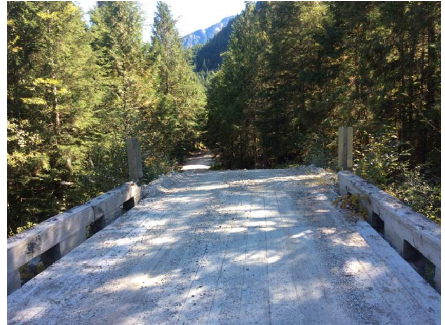
Right approach viewed from bridge
