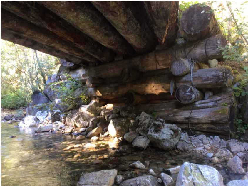
Left Bank Abutment when facing downstream
